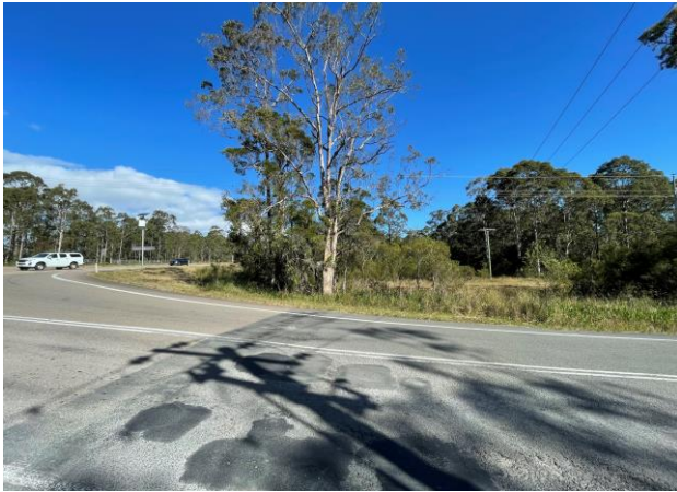
Photo 1 Corner of Italia Road and Pacific Highway damaged bitumen
